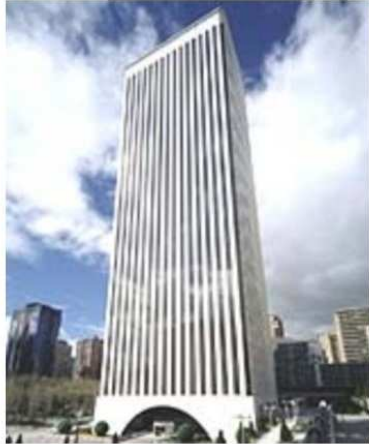
Picasso Tower (Madrid) Capacitor banks + 4 active filter APF
